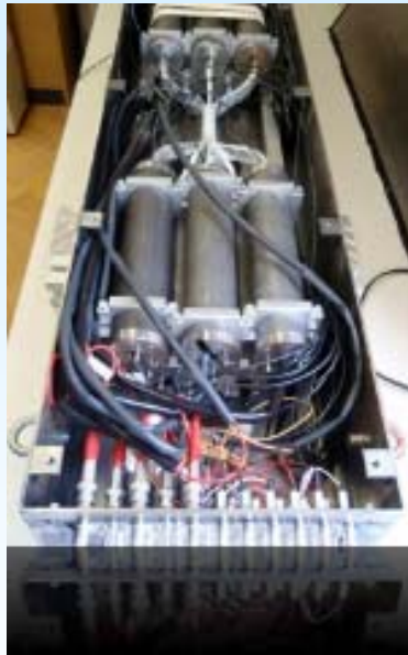
iron tubes and box for magnetic field shielding
